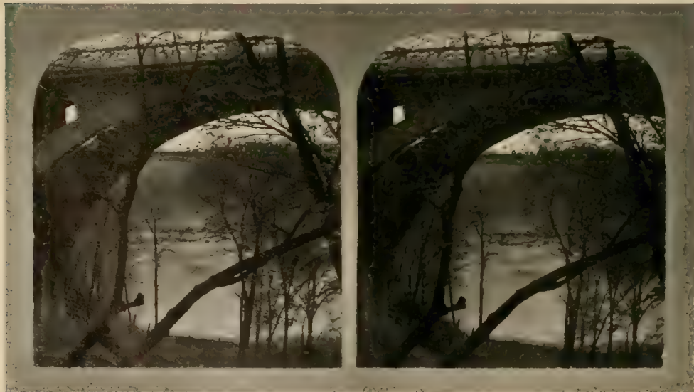
LAKE STREET AND BOULEVARD BRIDGE BETWEEN ST. PAUL AND MINNEAPOLIS By A. T. HUDELSON 568
